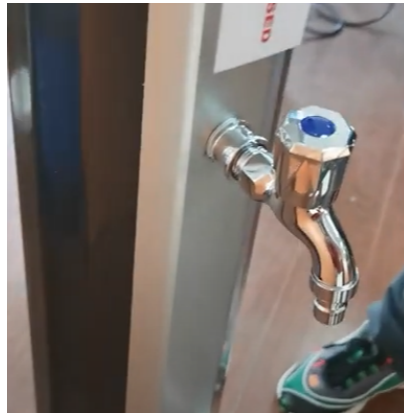
Screw in the faucet piece. Make sure the spigot part where water comes out is facing downward.
