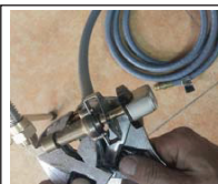
Install gas pipe.
