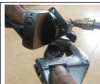
Remove propane pipe
